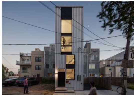
The 1,250 square foot single-family home glows at each of its five levels. While mindful of setbacks, it fills the site boundaries to achieve an elegant but efficient form.
