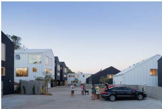
The multiunit buildings of the Blackbirds complex cluster around a shared courtyard and parking area.
