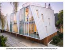
Photo: Buckner Architects
